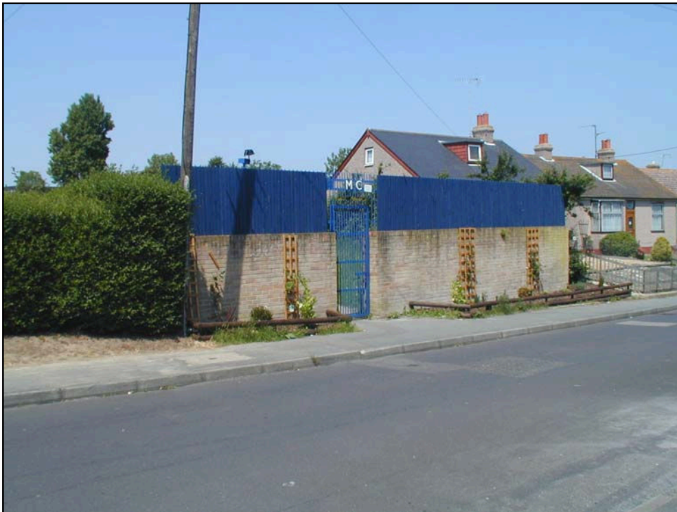
View looking north-westwards across the Minster College entrance on Parsonage Chase (taken when fence erected in 2006)
